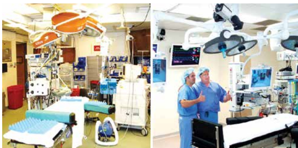
Fig. 2: Operation theater before and after integration
